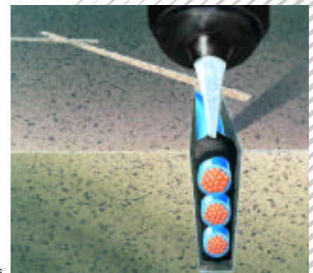
4. Fill sawcut with 3M ® Detector Loop Sealant.
